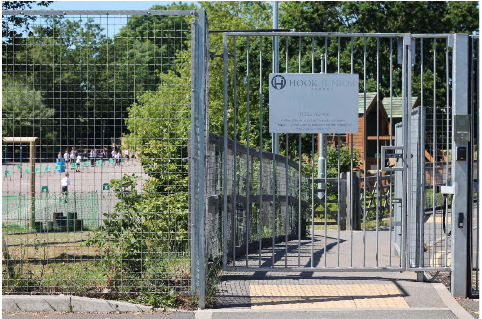
Access from the Community Centre Car Park
